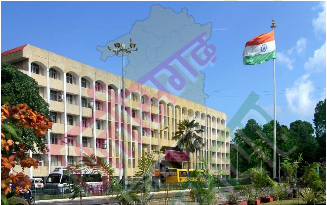
Administrative Block, JIPMER Puducherry
